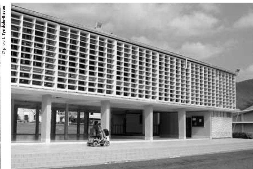
Fig. 5. University of the West Indies, part of Registry building
