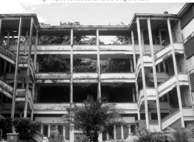
Fig. 4. Lycée Schœlcher, catwalks and flights of stairs
